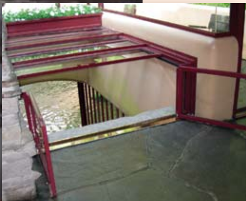
The hatch leads directly down to Bear Run Creek. When opened, air from below would help cool the living room. There is a small platform at the bottom of the stairs where the Kaufmanns would sit and enjoy the scenery or wade in the creek.
